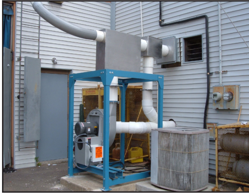
Outside Ground Instal
